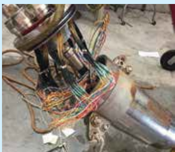
This is before the rebuild.
